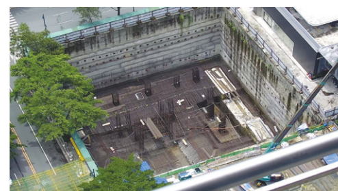
Rebar for Mat Foundation
