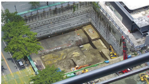
Completion of Bulk Excavation
