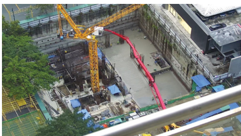
Completion of Mat Foundation
