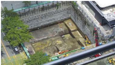
Completion of Bulk Excavation
