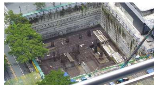
Rebar for Mat Foundation
