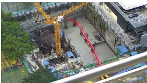
Completion of Mat Foundation
